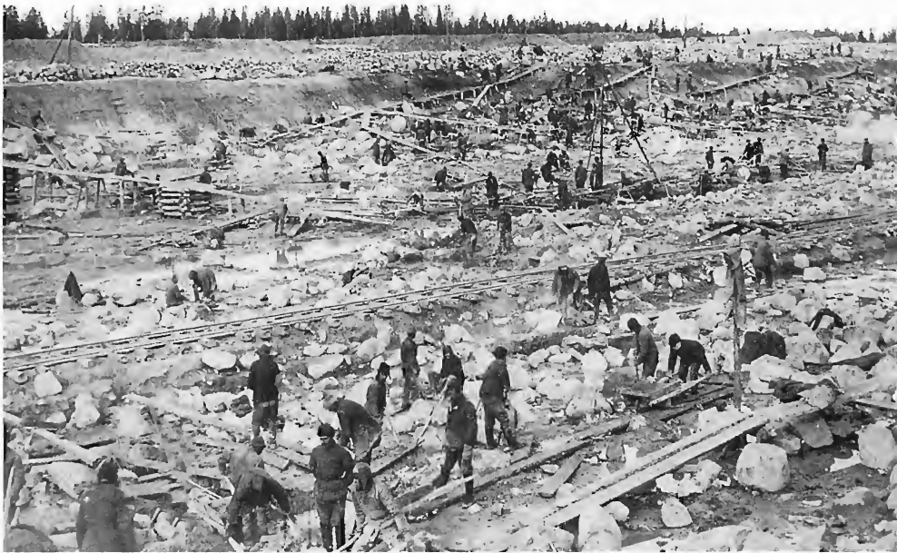
The construction site of the BBK, or Belomorkanal, the canal between the White Sea and the Baltic. This pharaonic project resulted in the deaths of tens of thousands of prisoners in 1932–33. The canal was opened amid great pomp by Stalin and his acolytes but proved to be useless. © Coll. Tomasz Kizny/Vu
