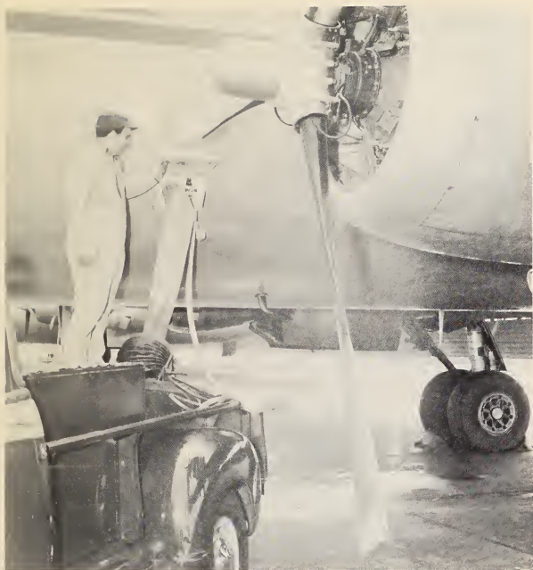
Removing toilet wastes from aircraft. (Note large, flexible sleeve which can be extended over hose to prevent spattering from defective valves.)
